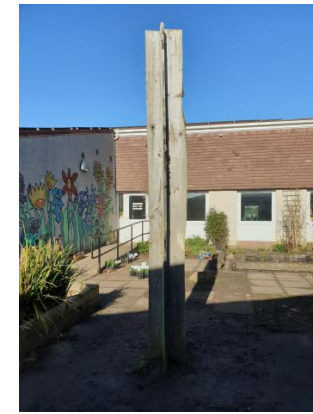
Central timber art feature
